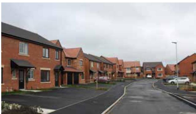
Figure 43: Example of a car/ parking dominated tertiary route, which would benefit from increased landscaping to soften its appearance, The Showfield
