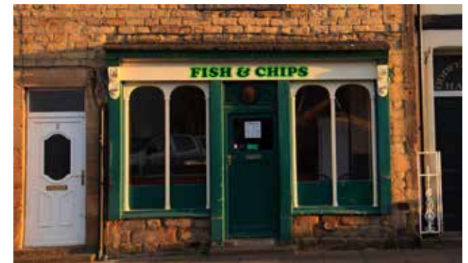
Figure 84: Traditional shop frontage enhances the streetscape
