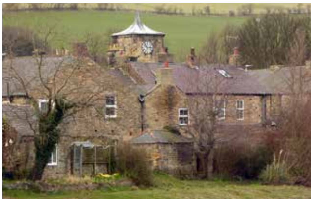
Figure 55: Chimneys create a varied roofscape
