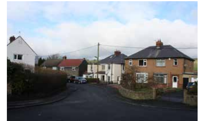
Figure 60: Semi detached properties at Whittis Crescent
