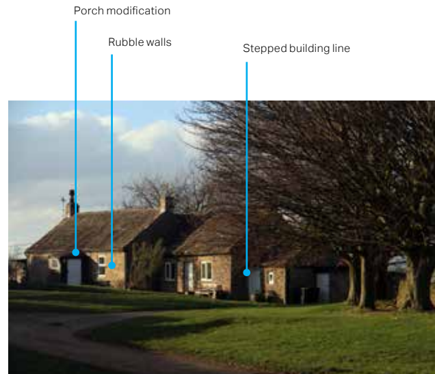
Figure 94: Low rise workers cottage in Elrington
