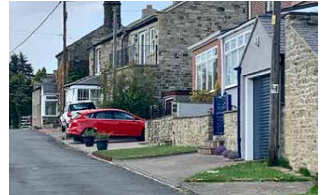
Figure 77: Front parking and garages at Heugh House Lane
