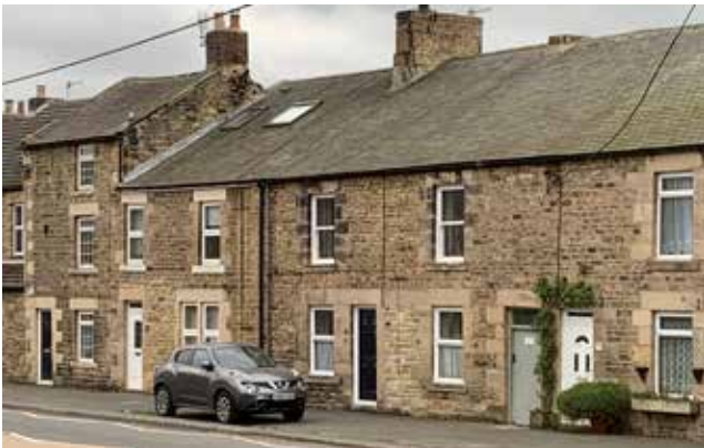
Figure 56: Terrace properties along Ratcliffe Road
