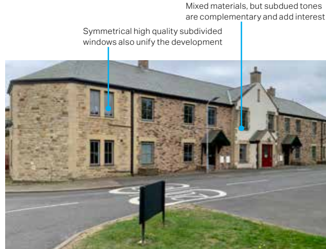
Figure 89: Old Foundry Yard Apartments, Strother Close
