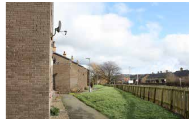
Figure 67: The staggered building lines at Langley Gardens are better suited to tertiary roads
