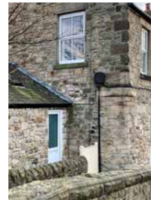
River stone rubble with quoins
