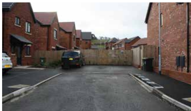
Figure 46: The cul-de-sac dominated layout of the Showfield Estate hinders pedestrian connectivity
