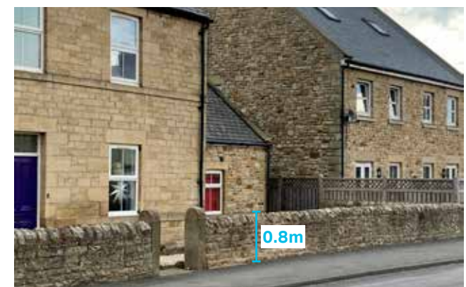
Figure 72: Positive example of low stone wall boundaries, with distinctive gateway pillars
