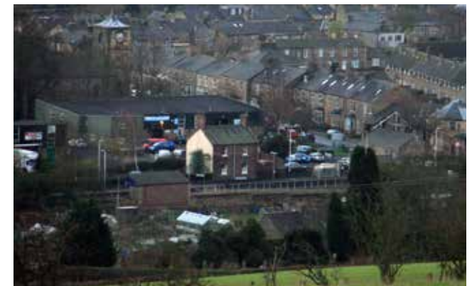
Figure 86: A small industrial area is located next to the railway station
