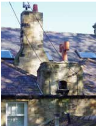
Chimney stack and skylights
