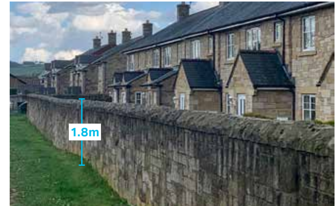
Figure 71: Taller boundaries can be used where there is a need for privacy eg. back garden facing on to road or side boundaries, although lower walls are often most suitable for street facing façades
