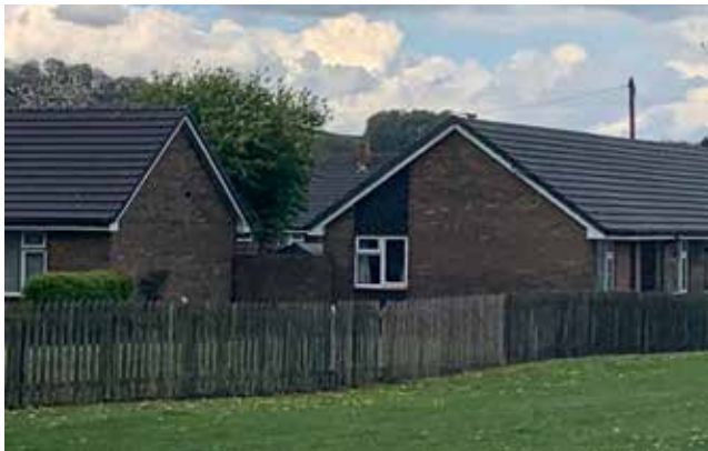
Figure 62: Bungalows at Greenwich Gardens
