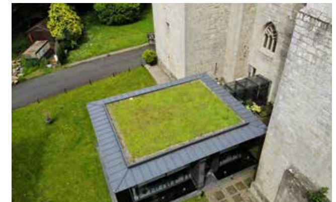
Figure 105: Good example of a modern extension with a sedum roof, to a Grade I listed building, Langley Castle
