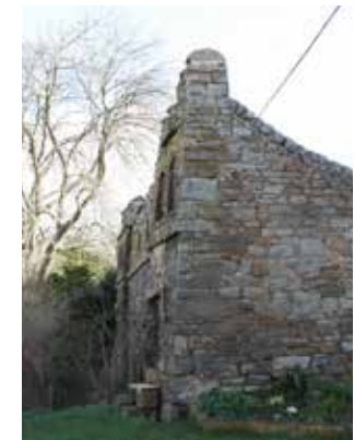
Figure 12: Castellated Wall at Shaftoe Terrace
