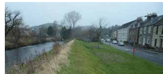
Figure 108: Good example of soft landscaped earth bund flood defence (outside of the parish)
