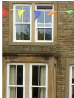
Wooden sashed windows
