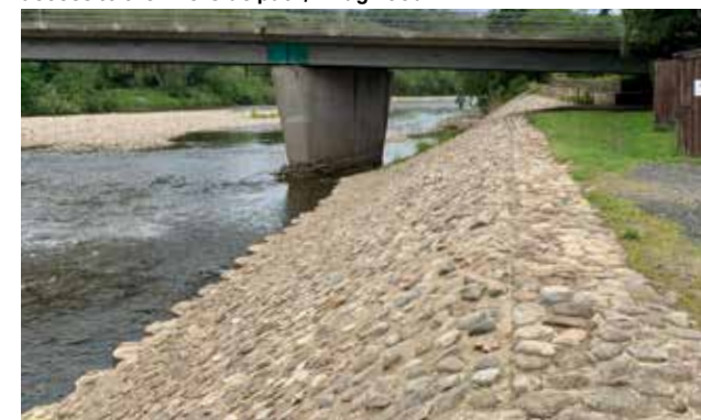
Figure 110: Existing engineered flood defences afford opportunities for further landscape enhancements
