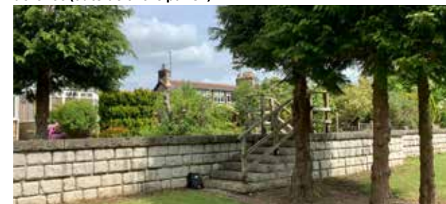
Figure 109: Good example of low flood walls with steps to provide access to the riverside path, Bridgwood
