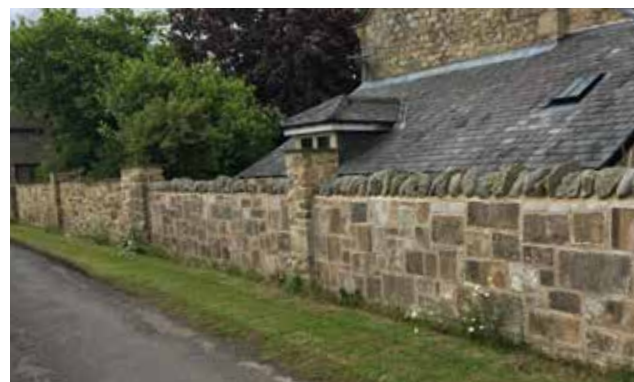
Figure 107: Good example of a flood wall constructed of natural stone, Lipwood
