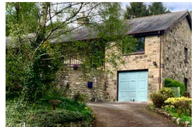
Figure 75: Built-in garage at property on North Bank
