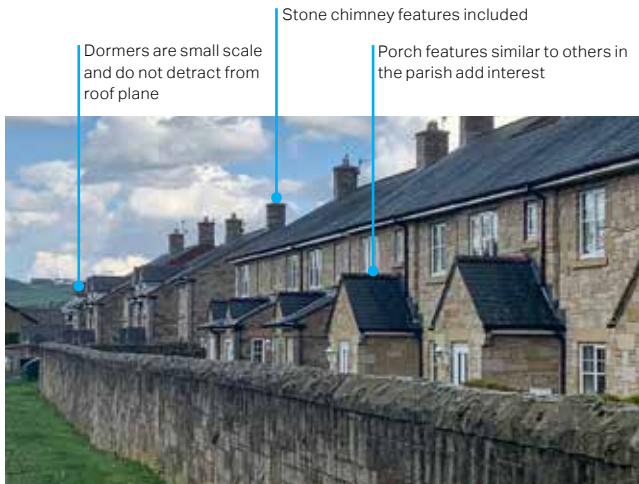
Figure 88: Properties facing Ratcliffe Road, Innerhaugh Mews
