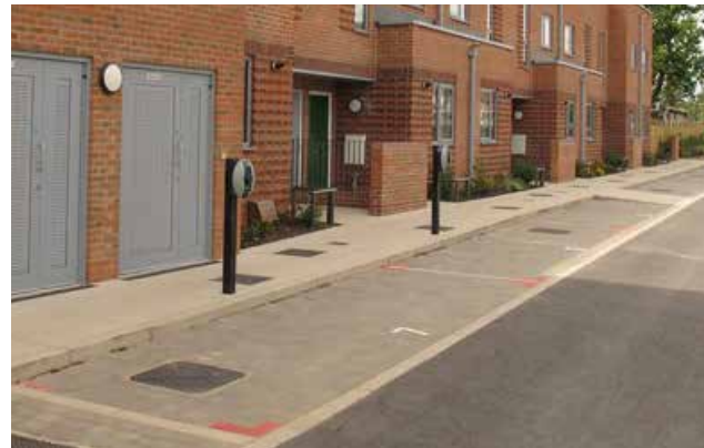
Figure 101: Electric charging points
