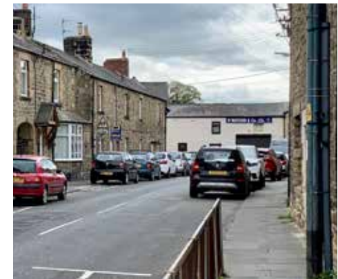
Figure 34: View along Shaftoe Street to Watson's Garage
