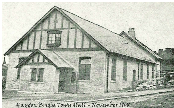
Haydon Bridge Town Hall - November 1908
